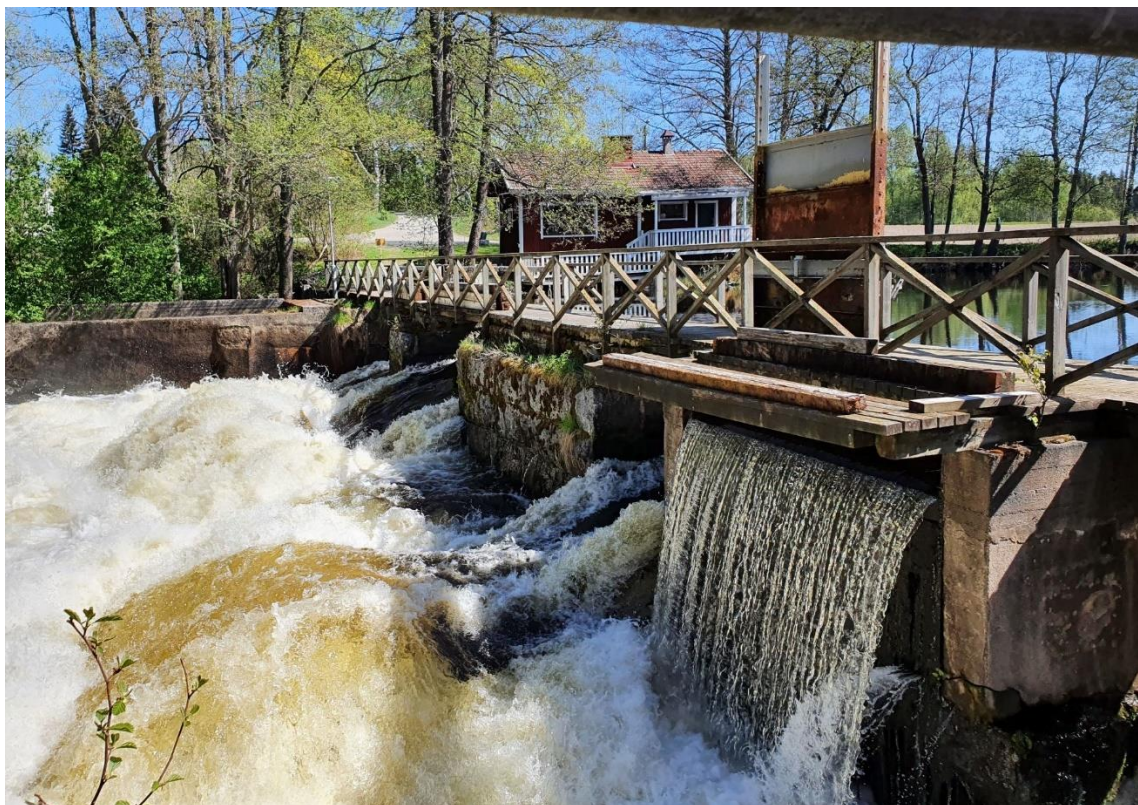
Virtaankoski hydro power plant dam to be demolished and River Tainionvirta 2022. Photo: own photo archives
