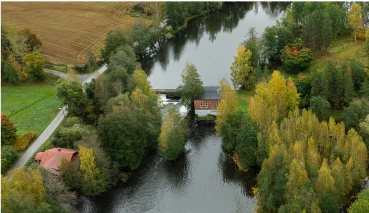
Virtaankoski power plant, dam and River Tainionvirta before the restoration on the 26 September.
